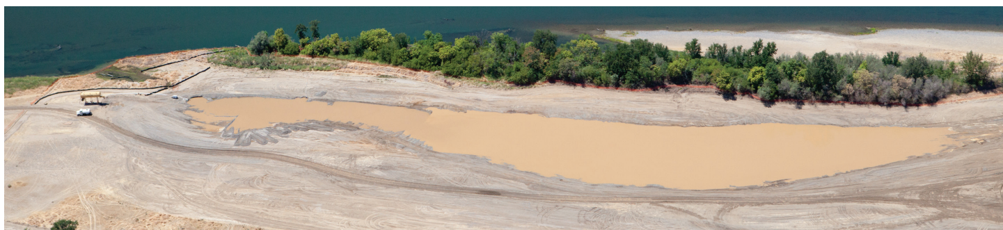
Overview of Construction at the Mitigation Site (June 2012)
